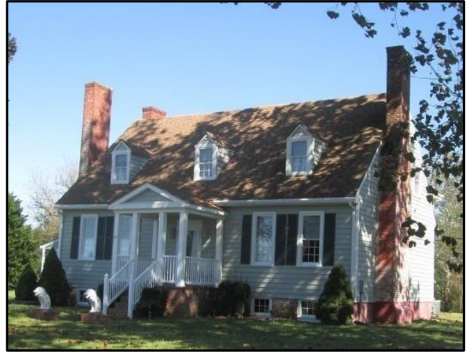
The rebuilt house between the remaining chimneys.
